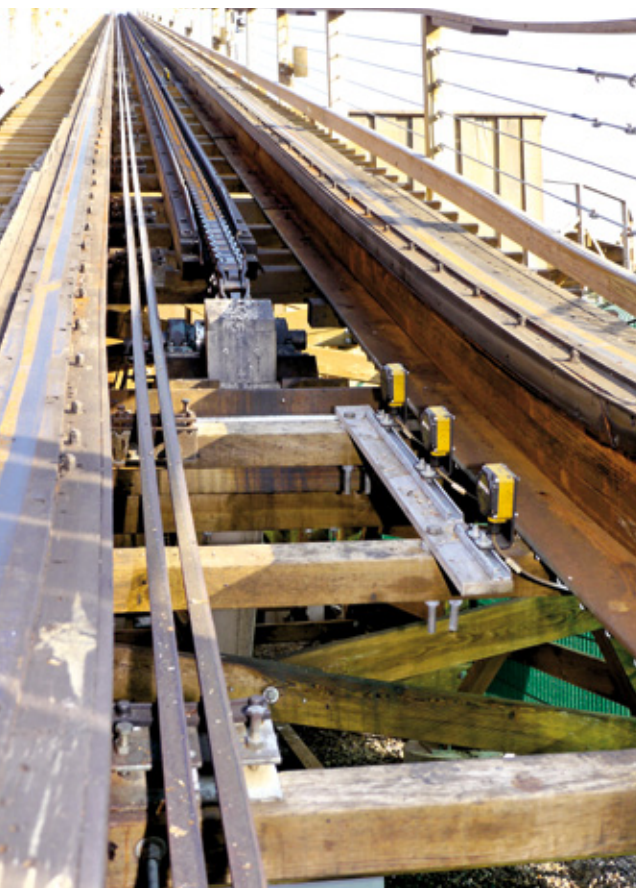
The train is detected by the uprox+ sensors over the entire lift phase
