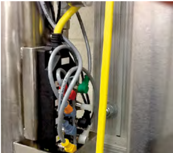
Anyone can connect these color-coded cables correctly to this junction box
