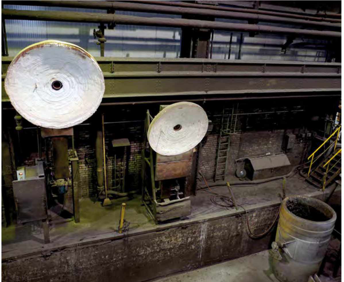
Gas burner XXL: The ladles (right) weighing several tons are heated in front of the white gas burners
