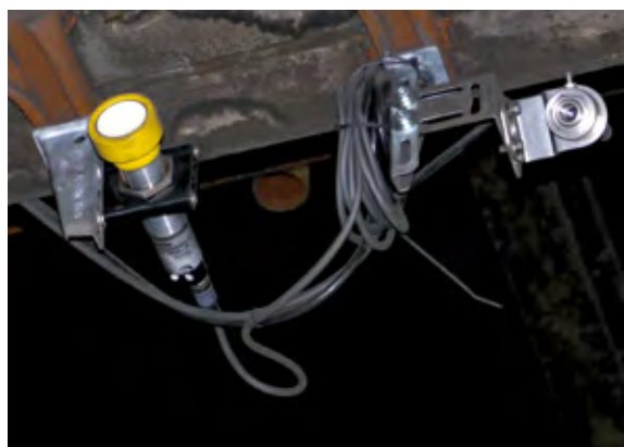
The ultrasonic sensor triggers the temperature measuring of the infra-red sensor (left)
