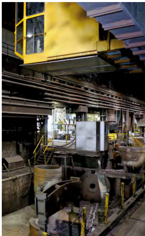
The crane driver in the control cabin (top right) sees all the temperatures of the relevant ladles
