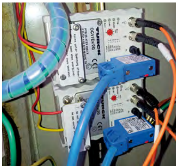
The optocouplers bring the Profibus signal from excom to the DCS via fiber optic cables
