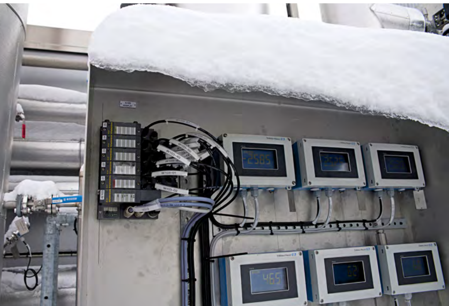
Keeping cool: With a temperature range up to -40 °C Turck's BL67 I/O system resists even Swedish winters
