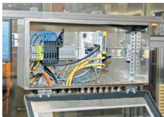
The BL20 gateway is programmable with CoDeSys and carries out the RFID communication
