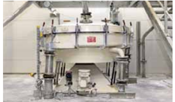
At its Burghausen site, WACKER is using Turck's BL ident RFID system for reliable detection in its tumbler screening systems in the dust Ex zone 22. Page 06
