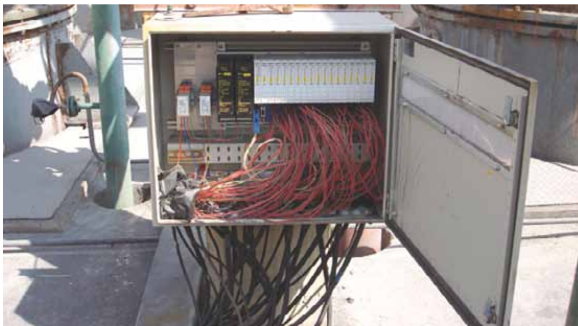
The excom remote I/O, consisting of power supply pack, gateway, I/O modules, and racks, can be configured using 24 V DC or 230 AC voltage
