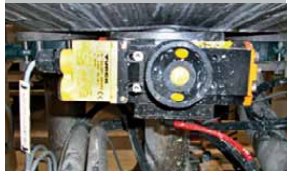
GAW Technologies in Austria has been relying on Turck dual sensors for position feedback signaling of butterfly valves and ball valves. Page 48
