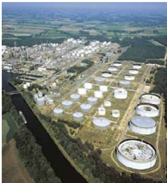
The BP Lingen Emsland oil refinery primarily produces gasoline and diesel fuels, jet fuel, light heating oil and chemical primary products
