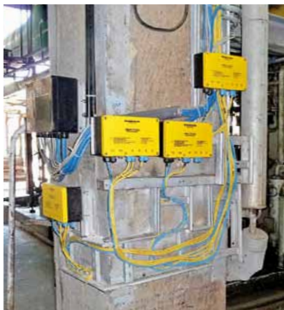
In hazardous areas, multi-barriers MBD49-T415/Ex with four intrinsically safe and isolated outputs are used
