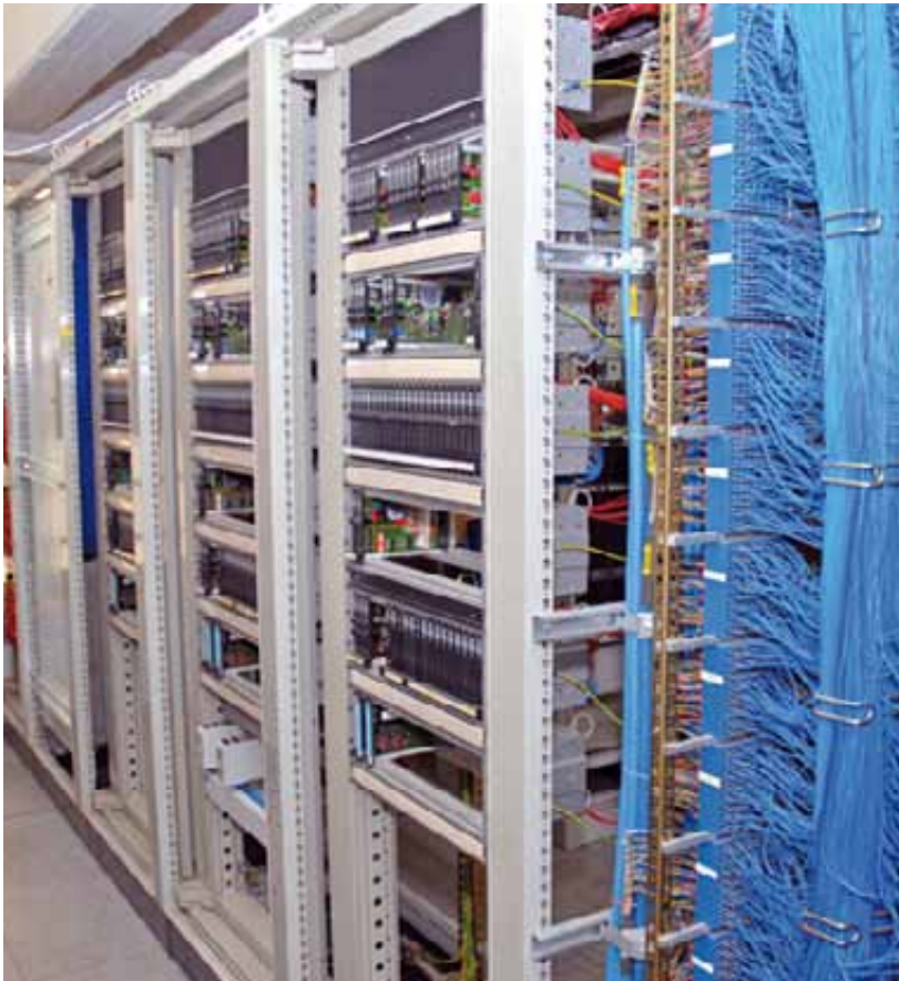
Since the modernization of the plant, the 19" rack (in the back) hosts two excom systems instead of the interface cards
