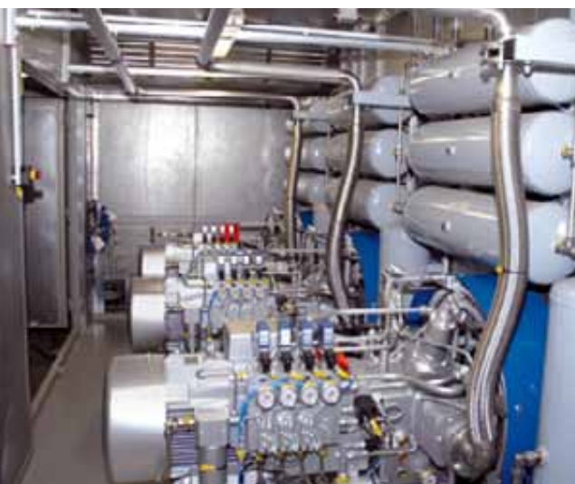
Up to four compressors compress the natural gas to the necessary 280 bar in several stages
