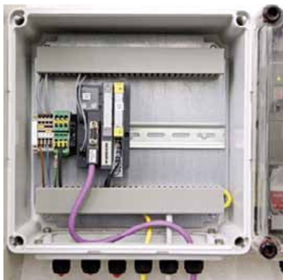
The screen data reaches the PCS7 process control system via Profibus and Turck's BL20 I/O system
