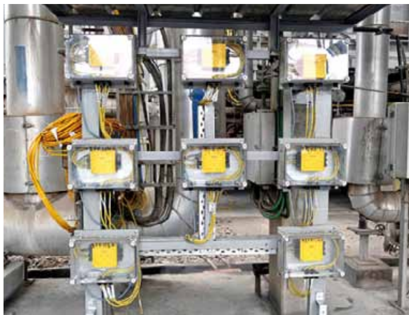
165 eight channel JBBS-49SC-T815 junction boxes from Turck guarantee a safe connection between the field devices and the DPC-systems
