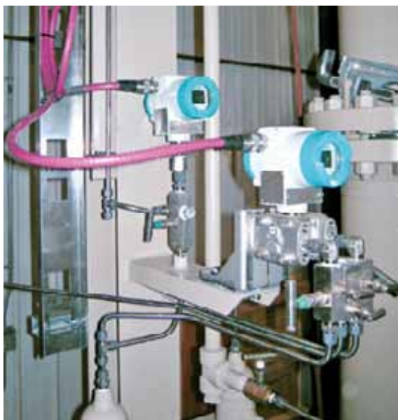
The instruments are connected to the junction block with armored single twisted pair cables
