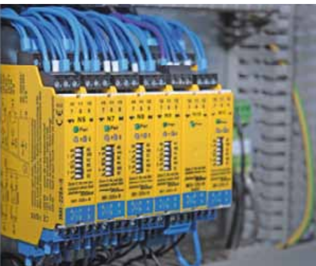
Intrinsically safe isolating amplifiers transmit the signals from the pressure sensors to the control unit
