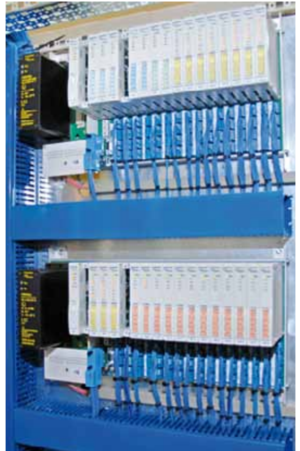
In only one weekend, EAB Automation installed the new excom systems into the 19" racks
