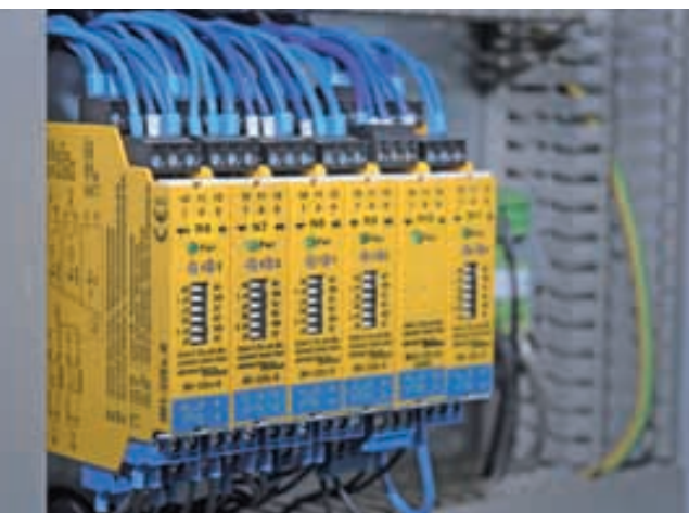
Intrinsically safe isolating amplifiers transmit the signals from the pressure sensors to the control unit
