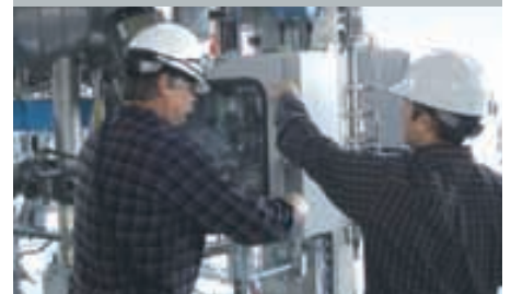
Intrinsically safe: excom remote I/O ensures reliable signals at Evonik Degussa North America Page 44
