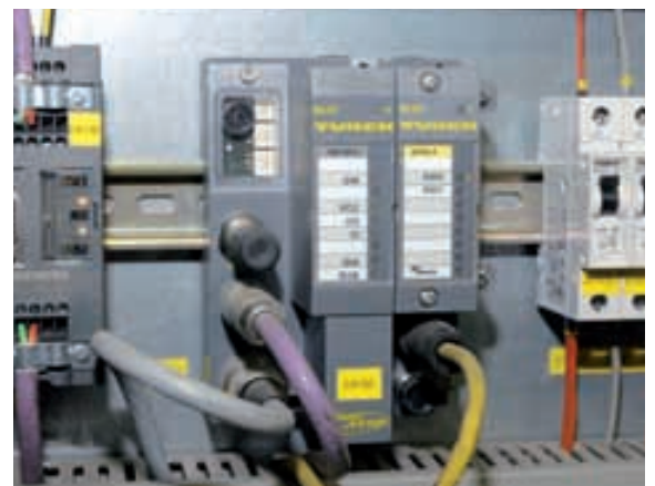
The signals are transmitted from the read-write heads to the control unit via the Turck I/O system BL67
