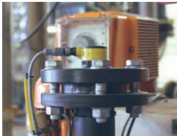
Ultrasound sensors from the type Banner T30UUPBQ monitor the filling level of the additives, which are required for water treatment
