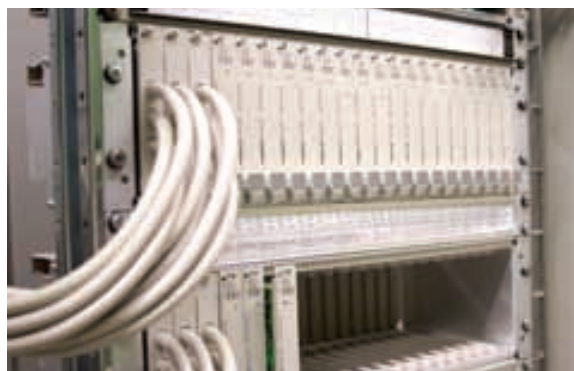
Infraserv Höchst uses interface technology in the 19-inch format for numerous measurements
