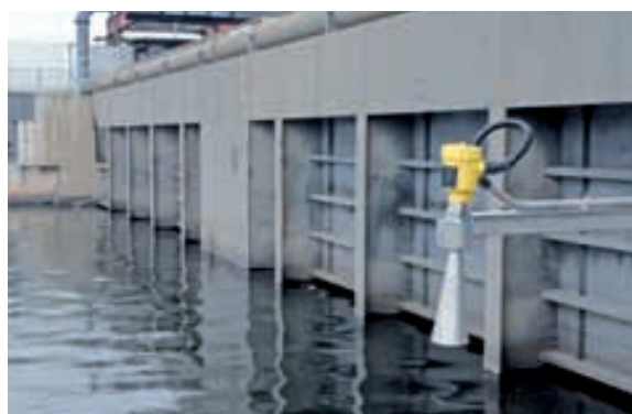
The waves of the radar sensors are reflected by the water surface, the elapsed time defines the level
