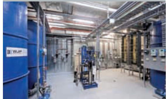
In Australia, WJP Solutions uses Turck's robust connection technology and BL20 distributed I/O system for their modular water treatment plants. Page 32
