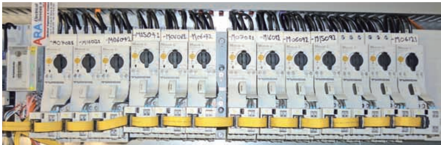
The motor starters, which are connected with a BL20 DeviceNet gateway, are installed in no time at all
